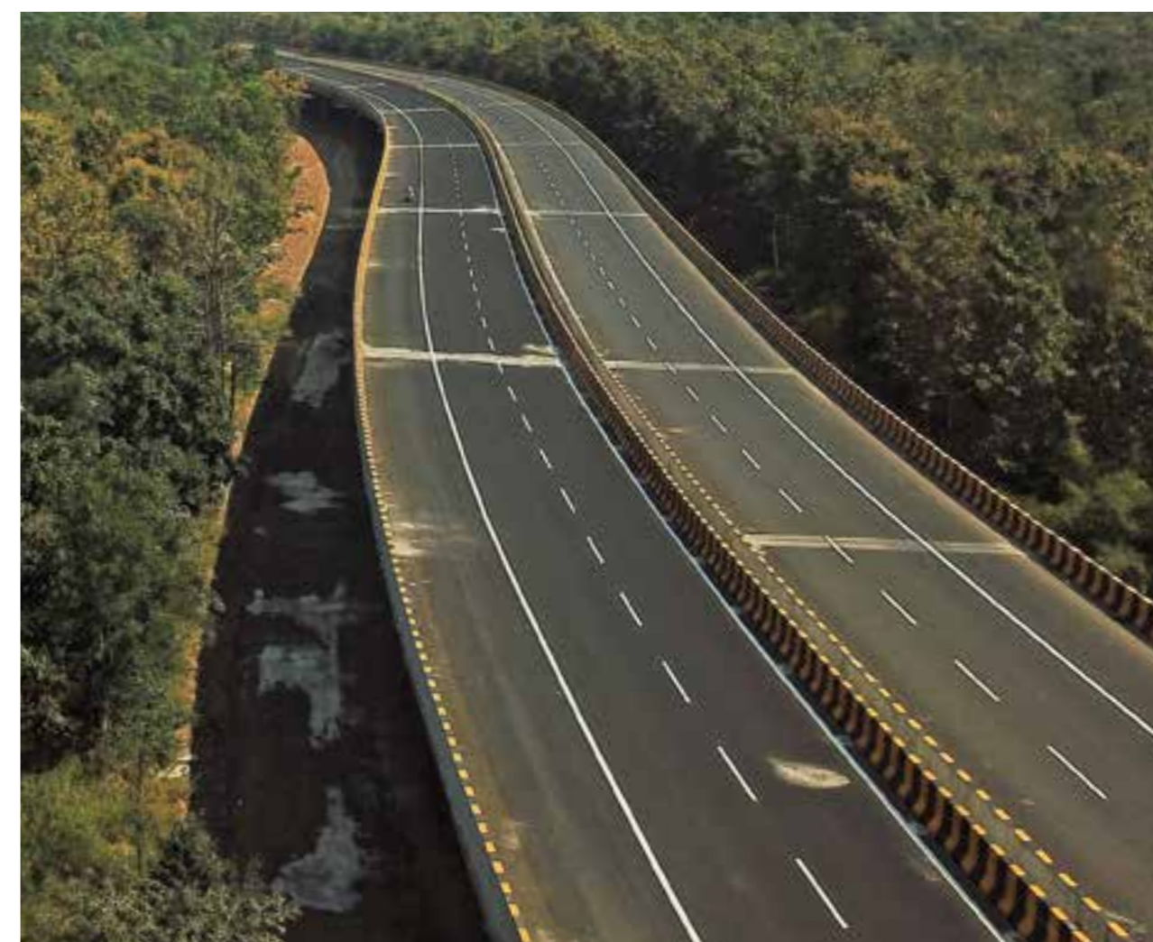
The elevated part of NH 7 (44) that houses the first functional underpass for wildlife © Milind Pariwakam/WCT
